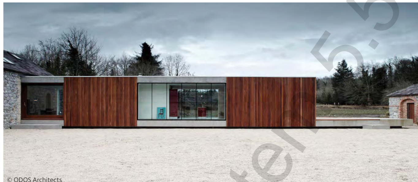
© ODOS Architects Ballymahon, by ODOS Architects
