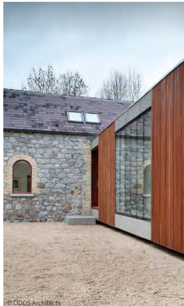
© ODOS Architects Ballymahon, by ODOS Architects
